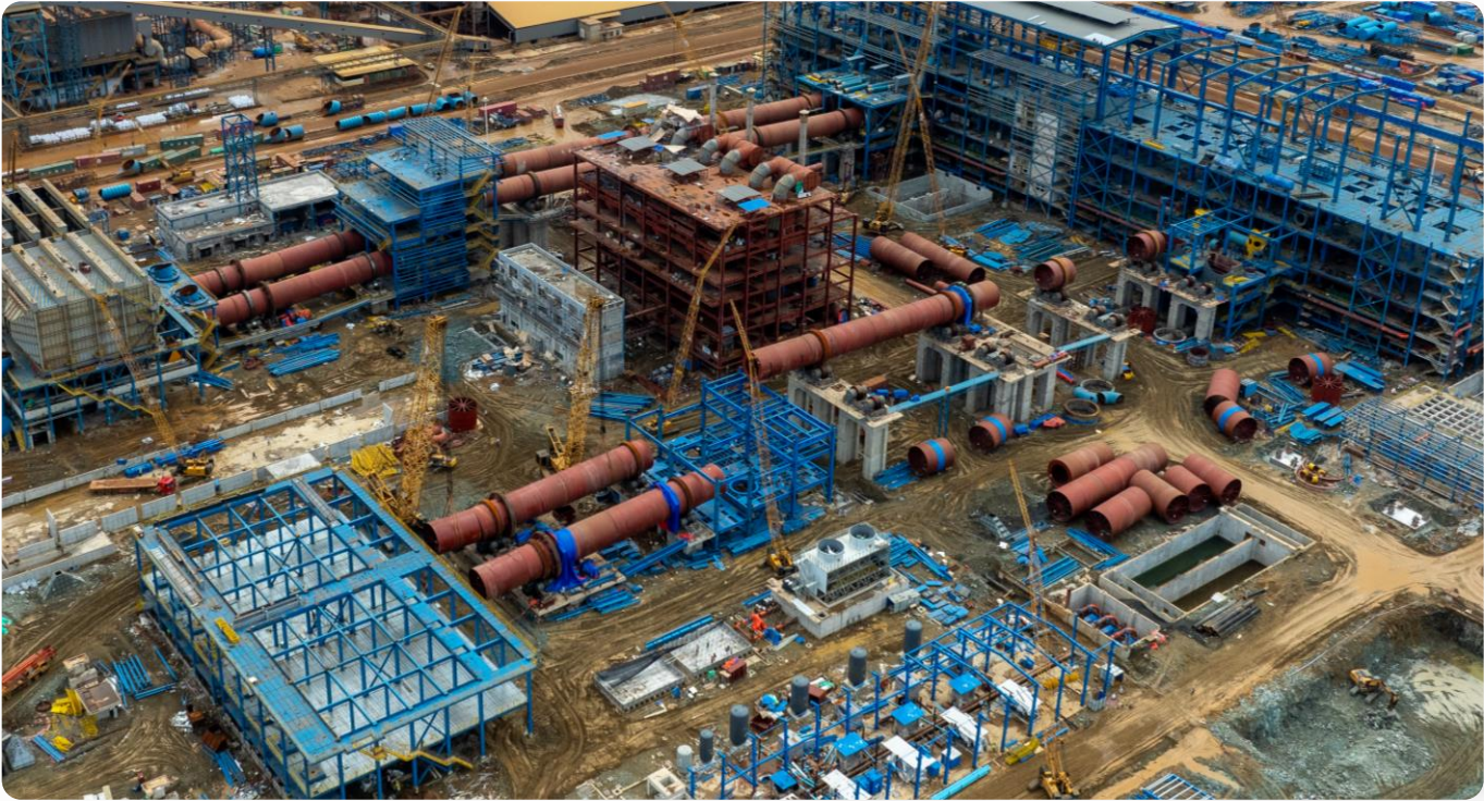
1 st phase progress – 4 lines
