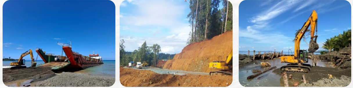
Jetty and road construction
